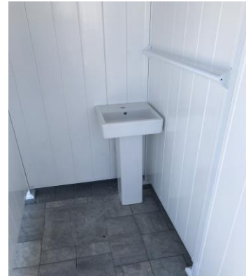
Interior Sink Install
